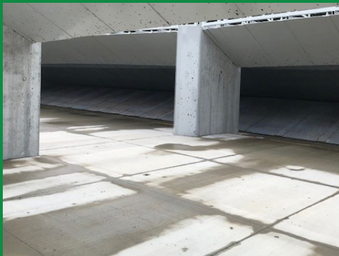
The front of the trap that funnels projectiles into the "mouth" of the trap – about a 3" horizontal gap that runs the entire length
