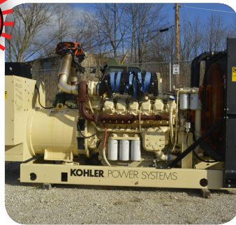
Kohler Generator Diesel, needs repair, 600 KW $7,500
