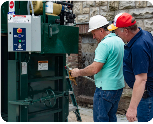
ACC's new baler was installed on May 26.
