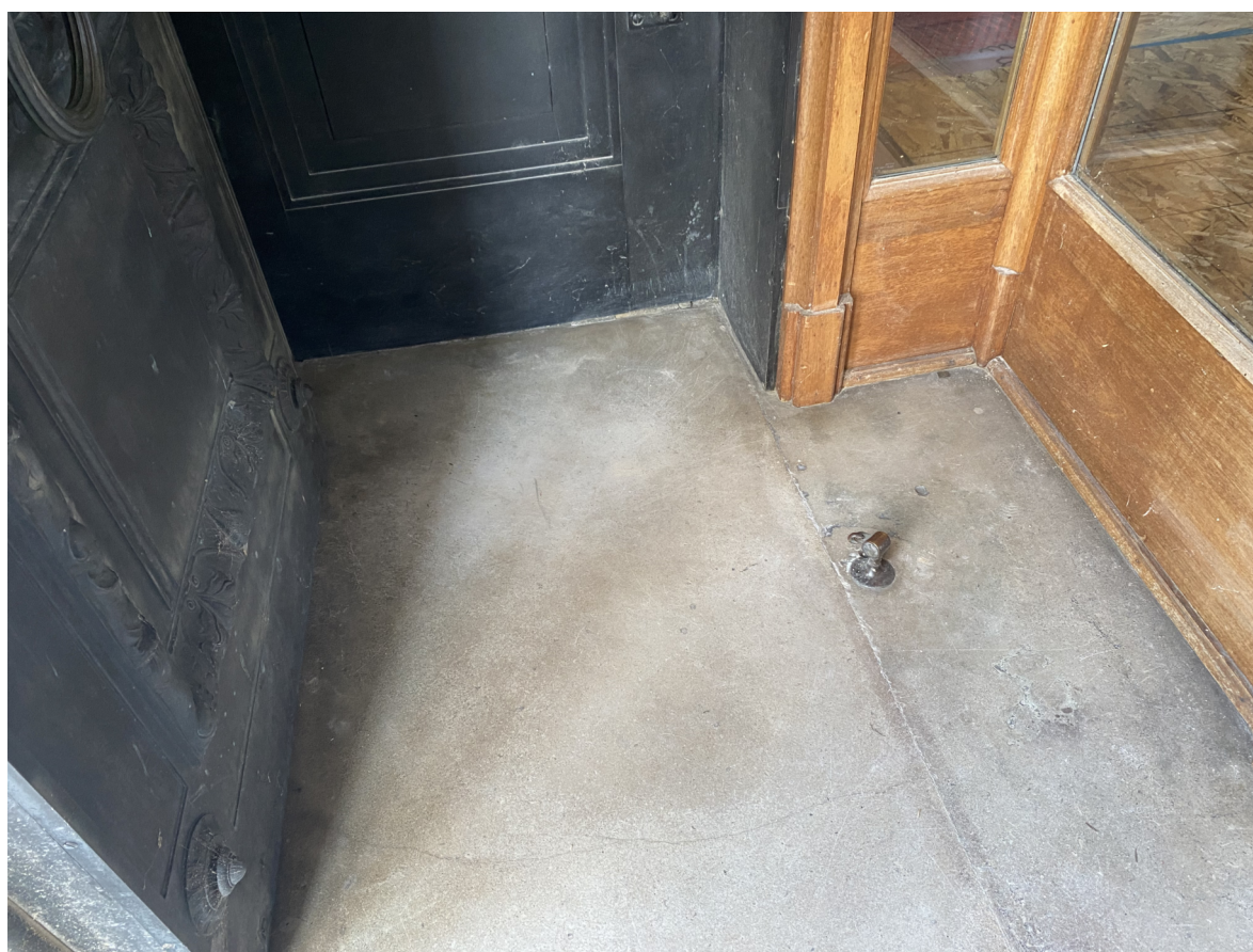
VIEW LOOKING WEST AT BASE OF CENTER VESTIBULE
