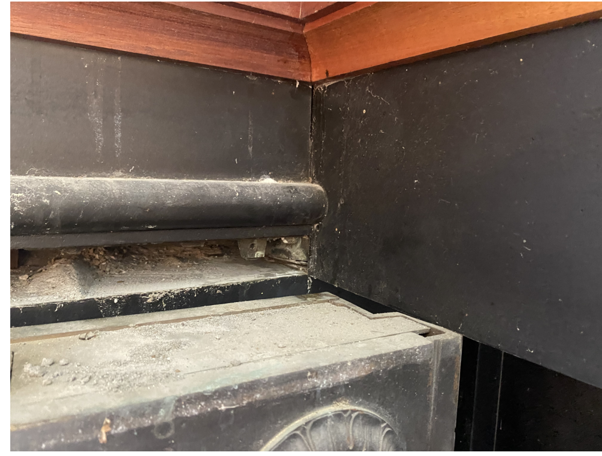
SOUTHWEST TOP INTERIOR CORNER OF CENTER VESTIBULE
