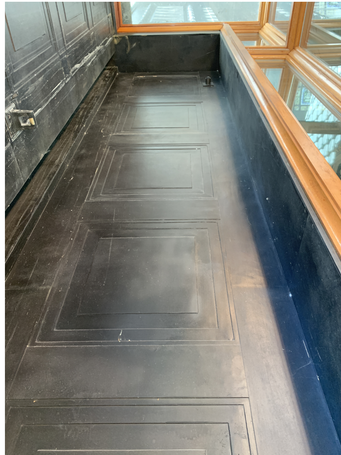
VIEW LOOKING UP WEST SIDE OF CENTER VESTIBULE
