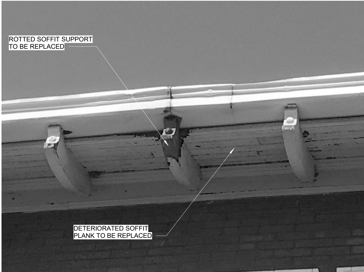
PHOTO 1 - DAMAGED SOFFIT FRAMING TO BE REPLACED
