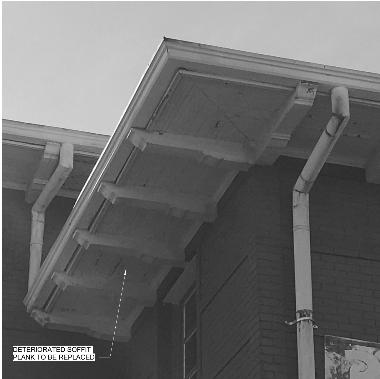
PHOTO 1 - DAMAGED SOFFIT FRAMING TO BE REPLACED
