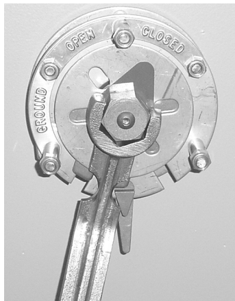
Figure 4A: Manual operation for motor actuator with quick disconnect coupling. Photo does not show motor actuator.
