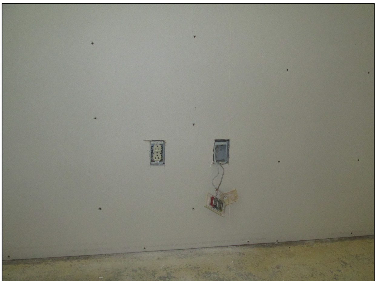
5 HDMI OUTLET + SPEAKER WIRES VISITATION RM NO SCALE
