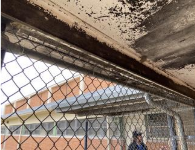
Photo 1 South End of Roof
