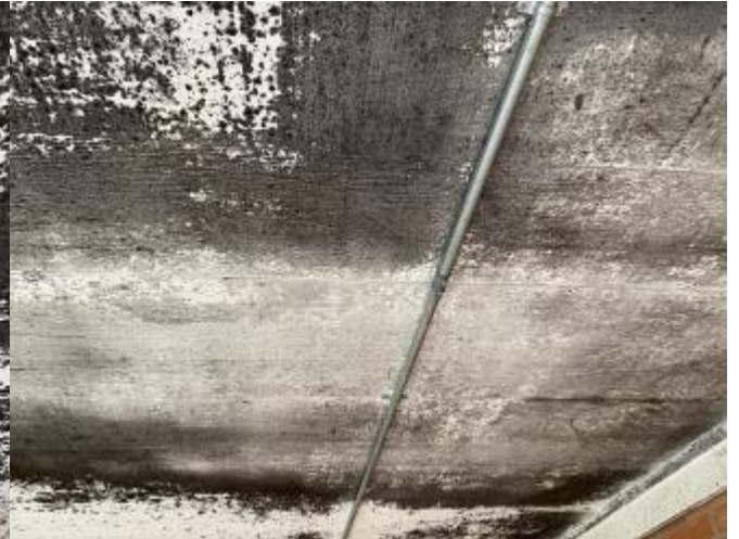
Photo 4 South End of Ceiling
