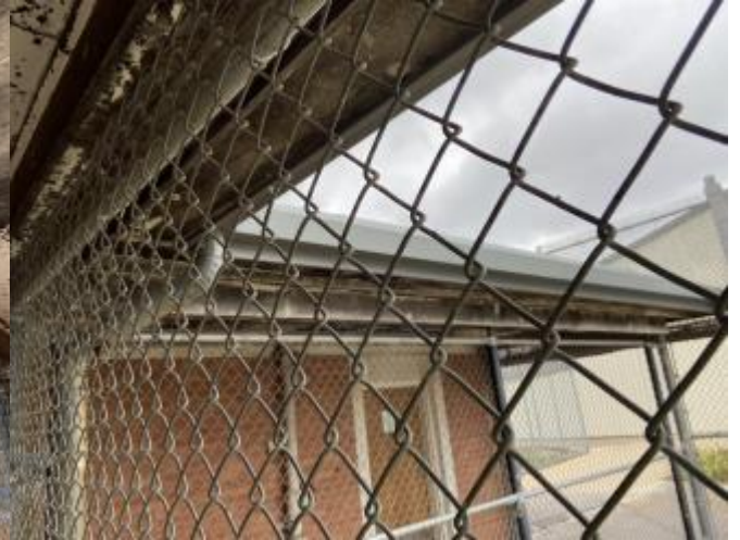
Photo 2 East End of Roof
