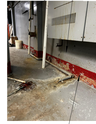
E SCRAPE FLAKING PAINT ON WALL SURFACE BELOW EQUIPMENT TO FLOOR. CLEAN AND PREPARE FOR NEW PAINT.
