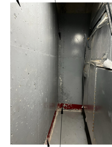
L SCRAPE FLAKING PAINT ON WALL SURFACE BELOW EQUIPMENT TO FLOOR. CLEAN AND PREPARE FOR NEW PAINT.
