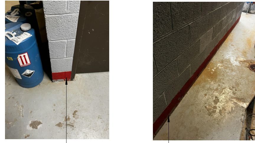
O CLEAN WALL BAND AND PREPARE SURFACE FOR NEW PAINT
