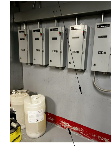
E SCRAPE FLAKING PAINT ON WALL SURFACE BELOW EQUIPMENT TO FLOOR. CLEAN AND PREPARE FOR NEW PAINT.
