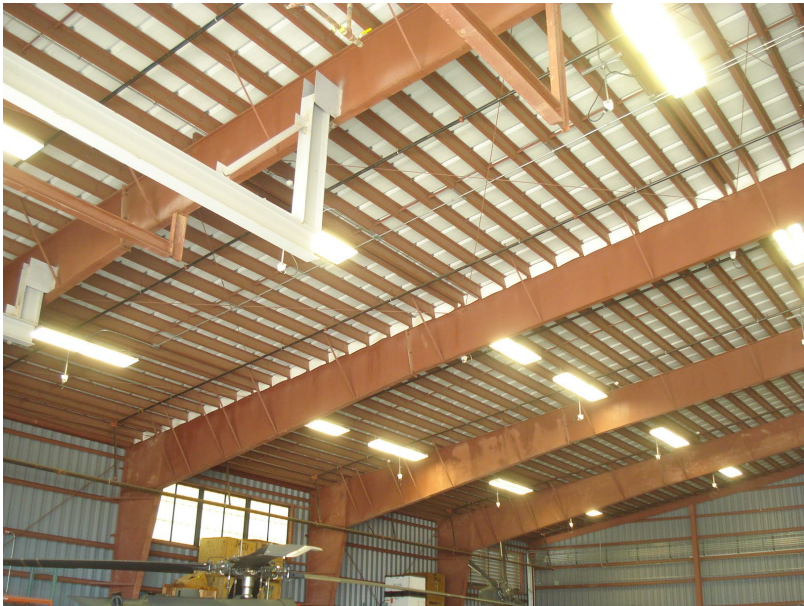
TYPICAL ROOF RIGID FRAMES/PURLINS "A"
