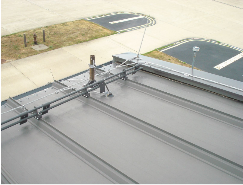
ROOF AT CORNER GRID H-6 "A"
