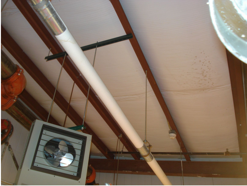
INTERIOR ROOF "B"
