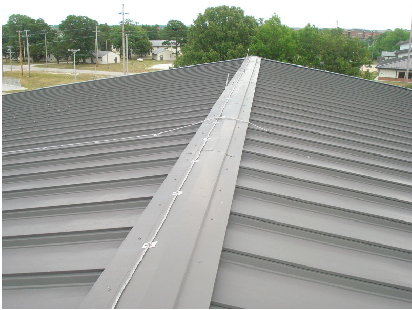
ROOF RIDGE "A"
