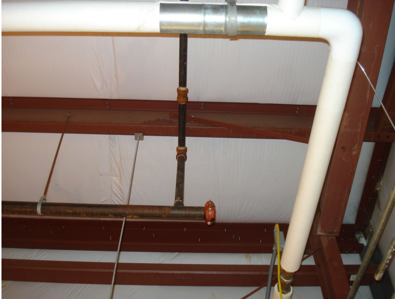
INTERIOR ROOF "B"
