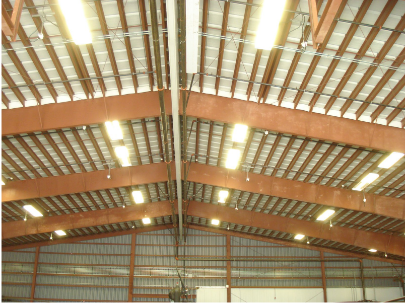
INTERIOR RIDGE "A"
