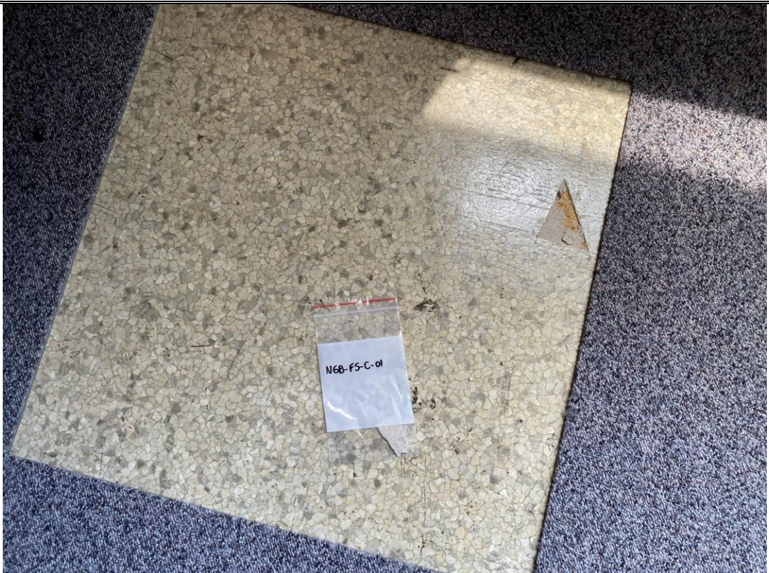
View of non-ACM floor sheeting, pebble pattern.
