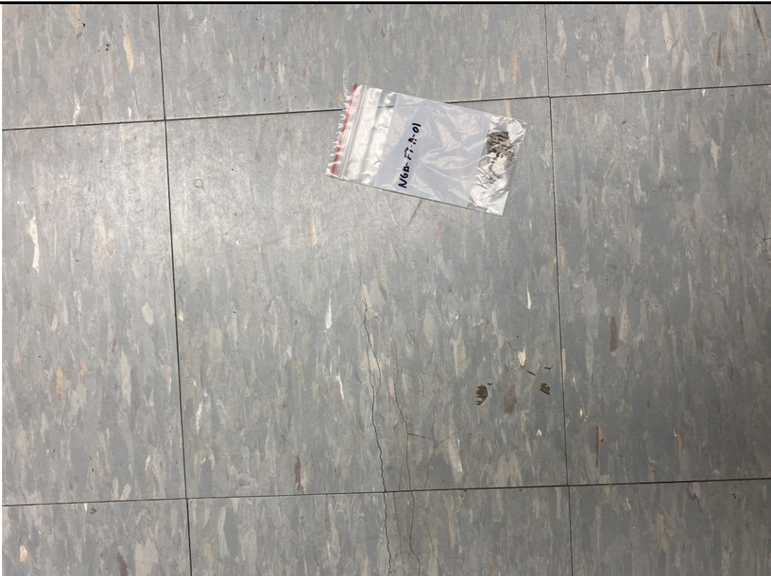
View of non-ACM 12"x 12" floor tile with non-ACM mastic.
