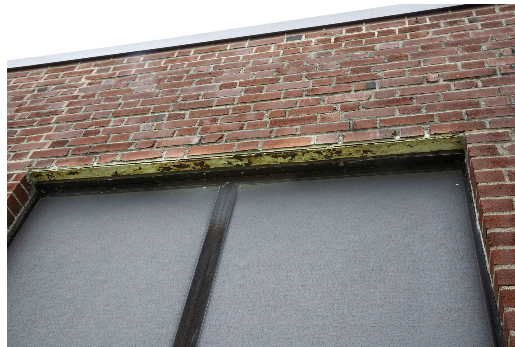
6 TYPICAL LINTEL CONDITION NTS
