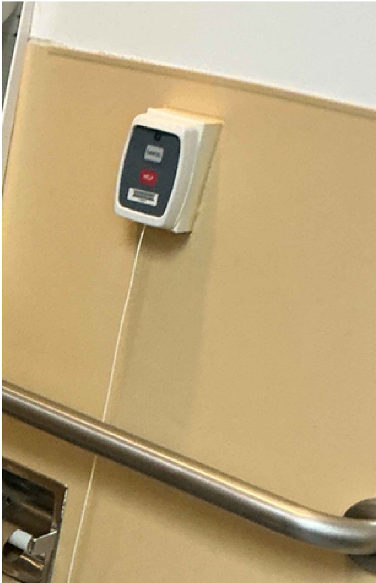
TYPICAL CURRENT PULLCORD STATION LOCATION
