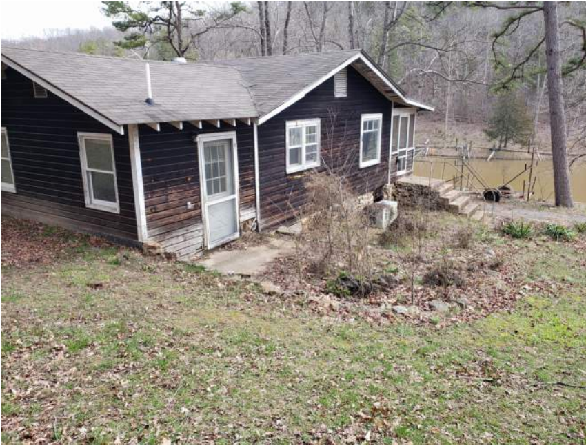
#5: FAMILY CABIN, EXTERIOR SOUTH WEST VIEW
