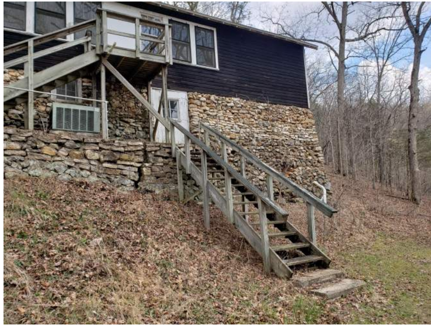
#5: LOWER DORM, EXTERIOR SOUTH VIEW
