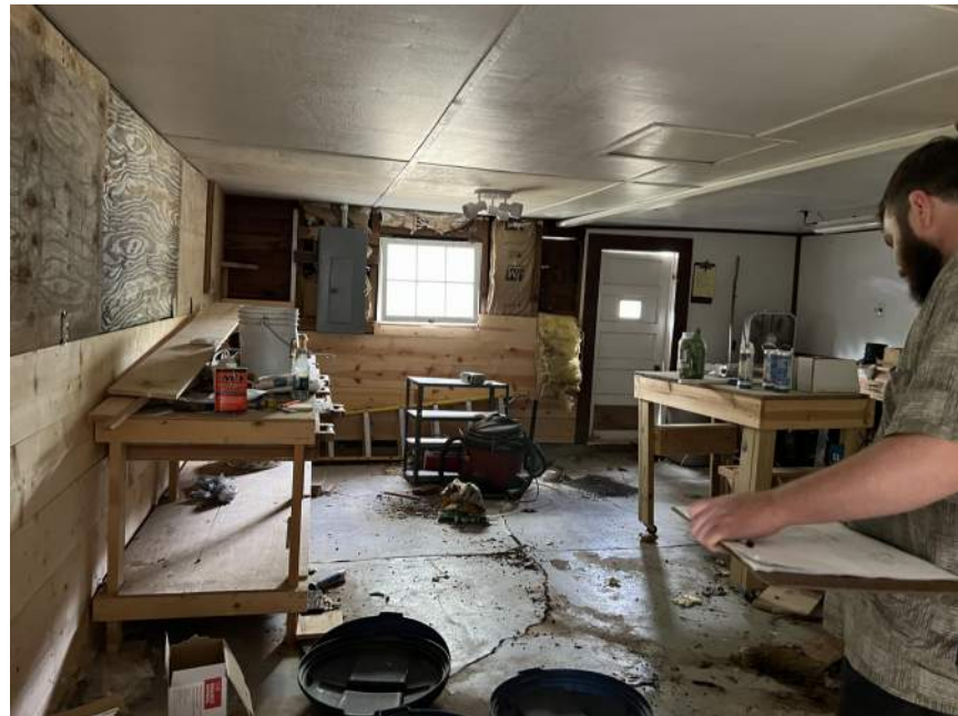
#1: BATHROOM BUILDING, INTERIOR
