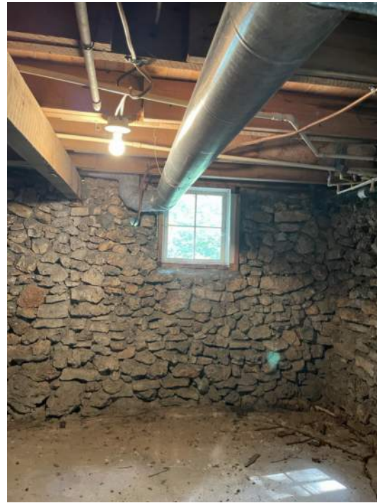
#2: LOWER DORM, BUILDING, INTERIOR EAST VIEW
