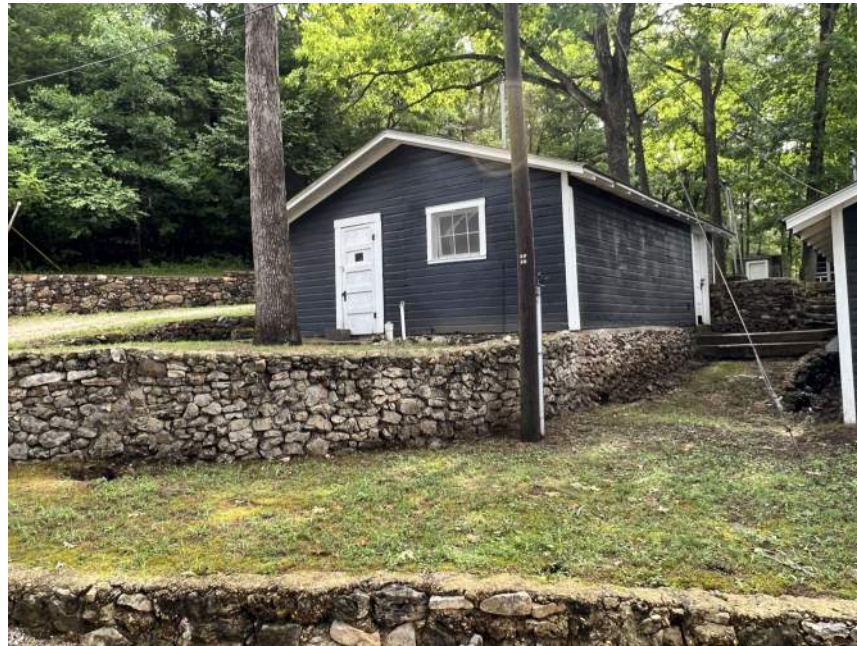
#2: BATHROOM BUILDING, EXTERIOR
