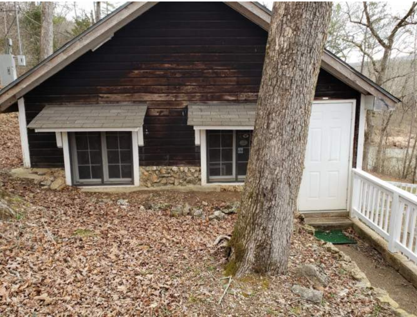
#3: GAMEROOM BUILDING, EXTERIOR ENTRY
