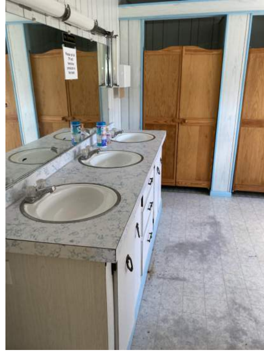
#9: LOWER DORM, INTERIOR RESTROOM VIEW
