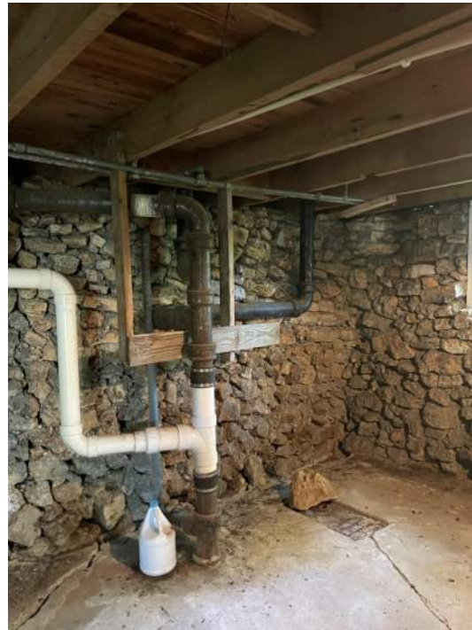
#1: LOWER DORM, BUILDING, INTERIOR NORTH VIEW
