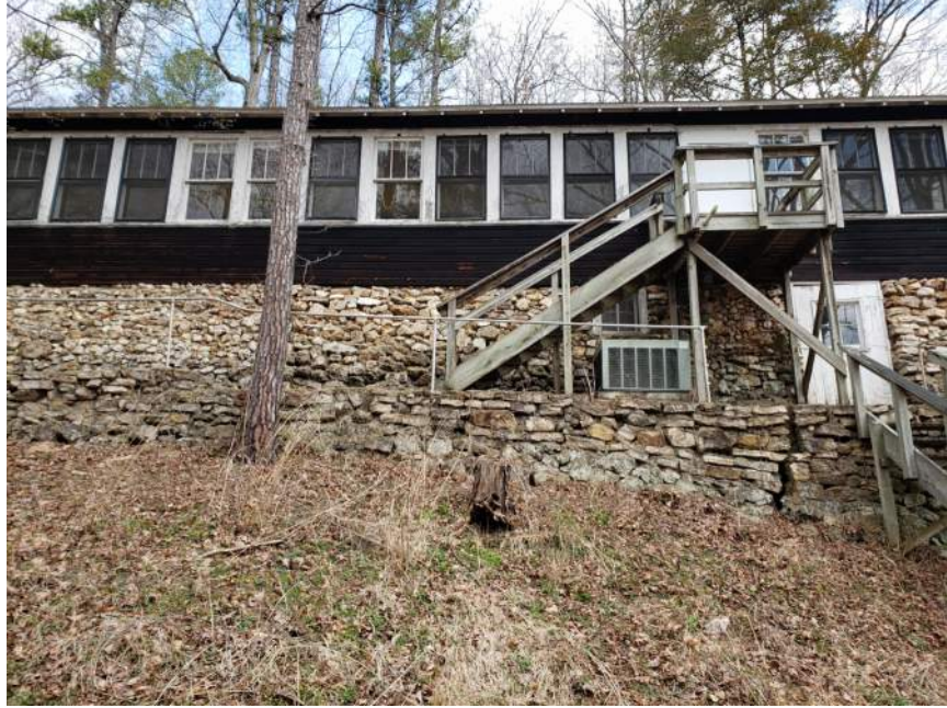
#6: LOWER DORM, EXTERIOR SOUTH VIEW
