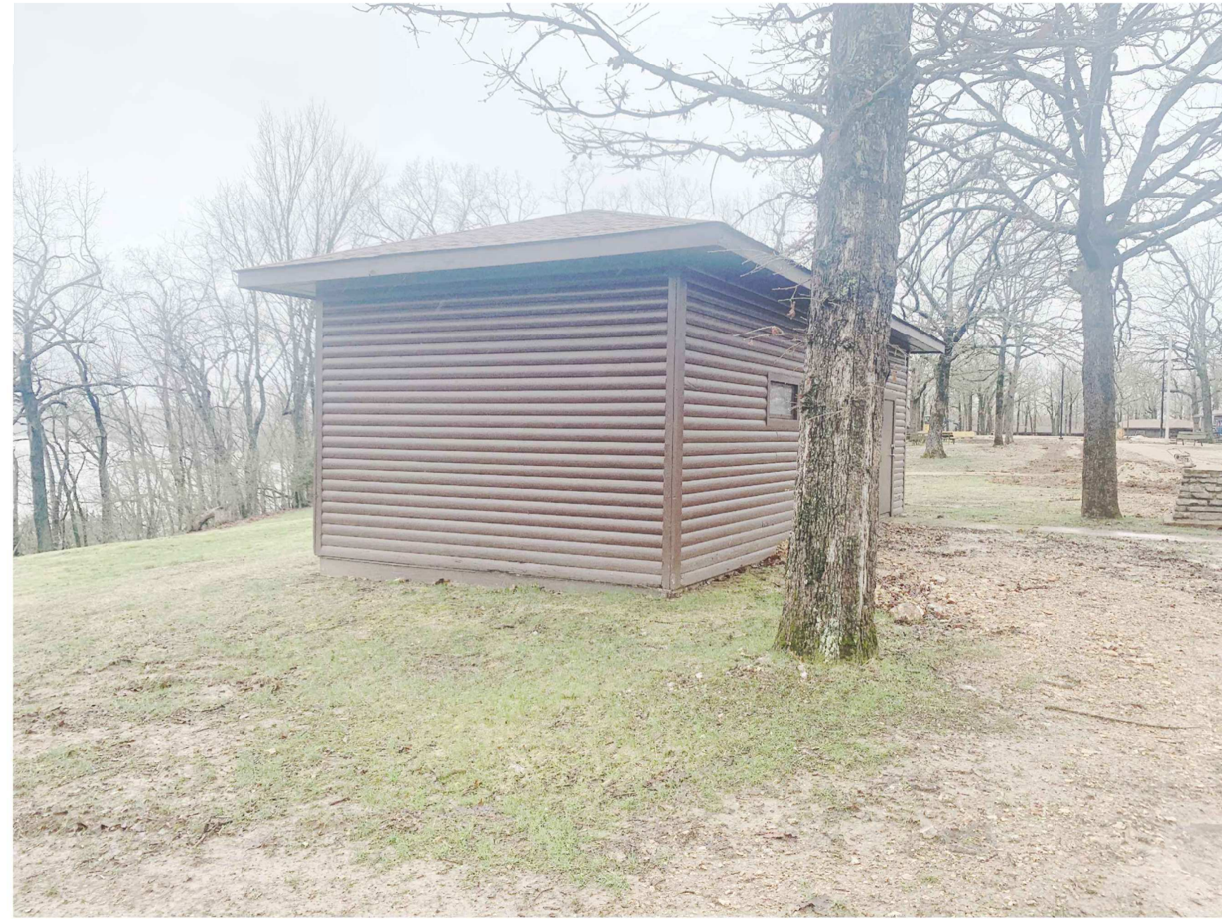
EXISTING TANK AND WELLHOUSE BUILDING
