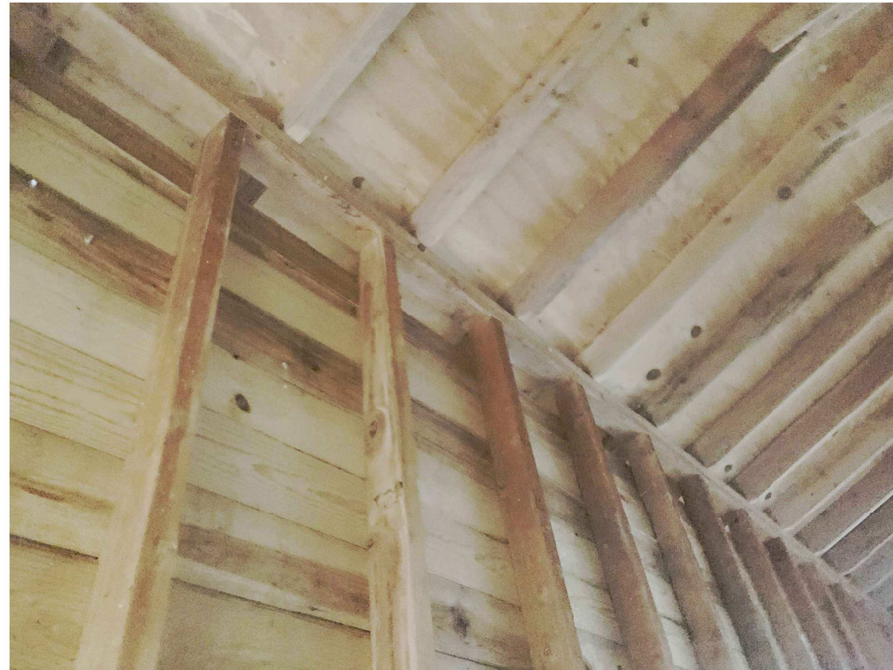
EXISTING ROOF FRAMING
