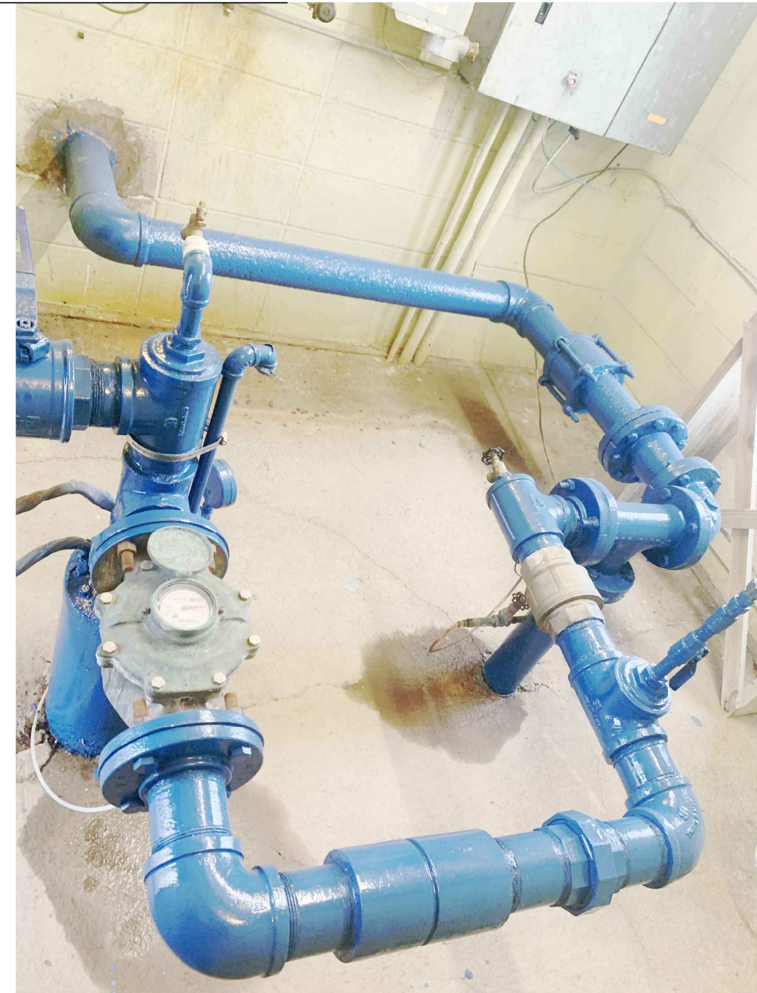
EXISTING WELLHOUSE PIPING
