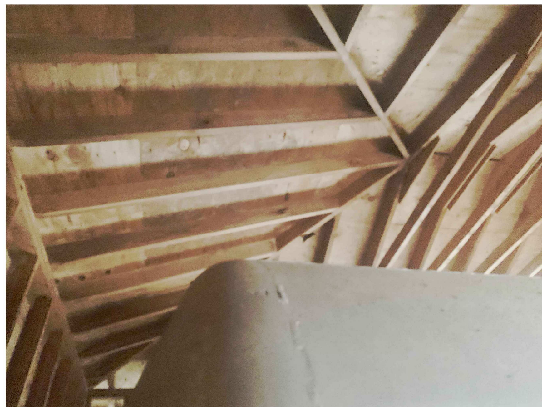
EXISTING ROOF FRAMING
