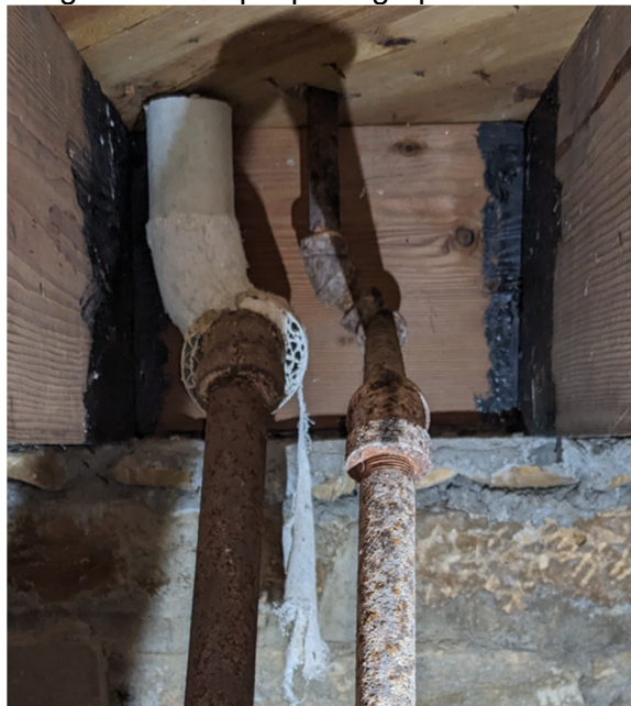
Figure 3.4 – ACM Insulation at Steam and Condensate Risers
