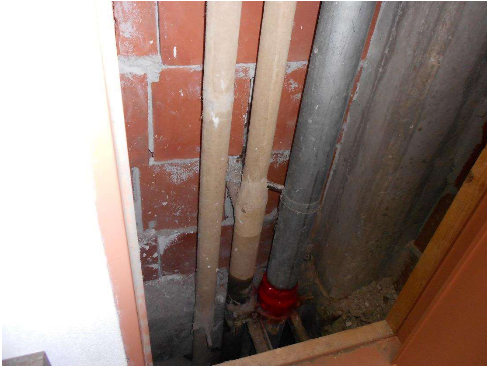
Figure 3: Bldg. 3, typical pipe chase
