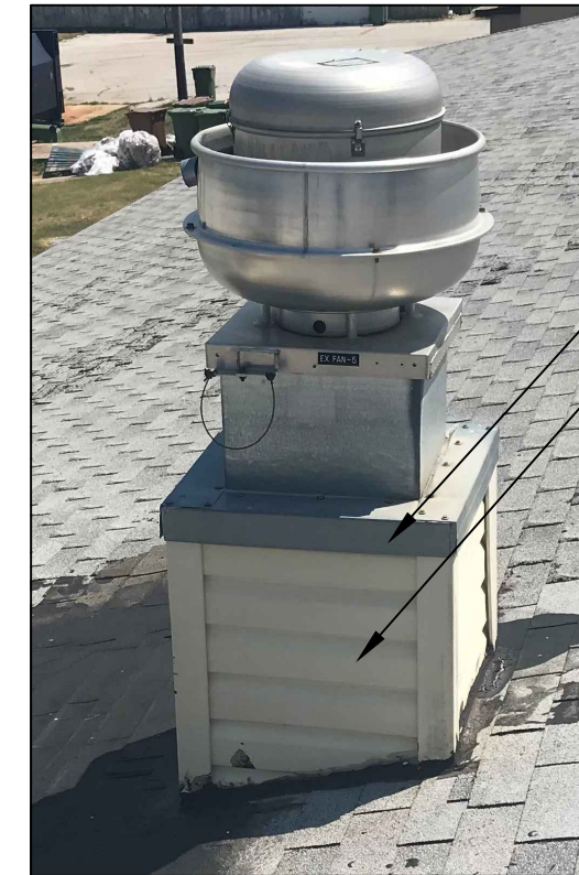
4 EXISTING EXHAUST PENETRATION REFER TO NOTES "K" AND "H"
