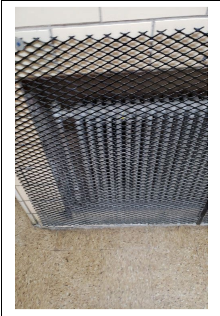
Photo 11. 254 - Black grate in hallway outside of Room 14-111
