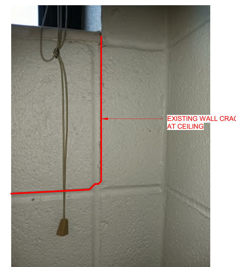
P5 SITE PHOTO 12" = 1'-0"
