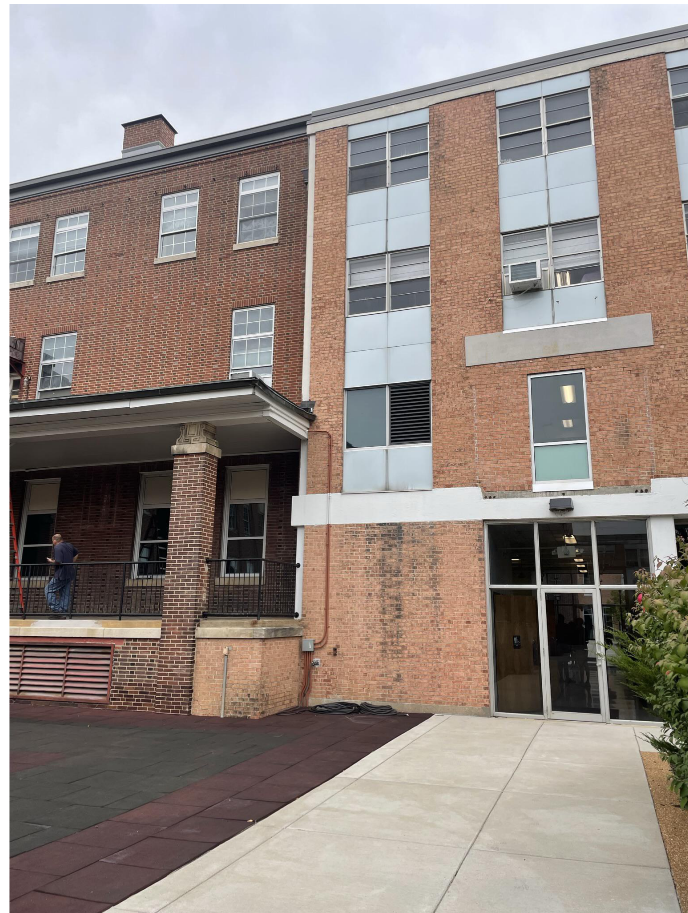
6 PHOTO OF EXISTING BUILDING G-003 1/2" = 1'-0"
