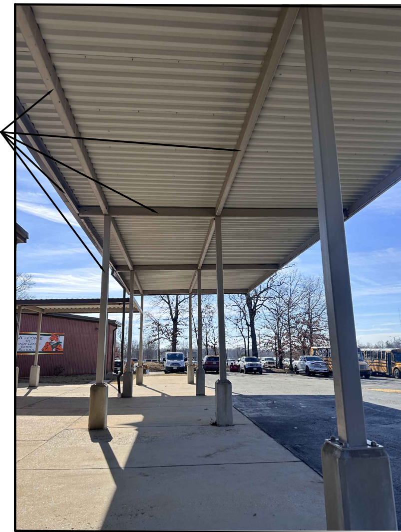
PICTURE NO. 1 - TYPICAL CANOPY
