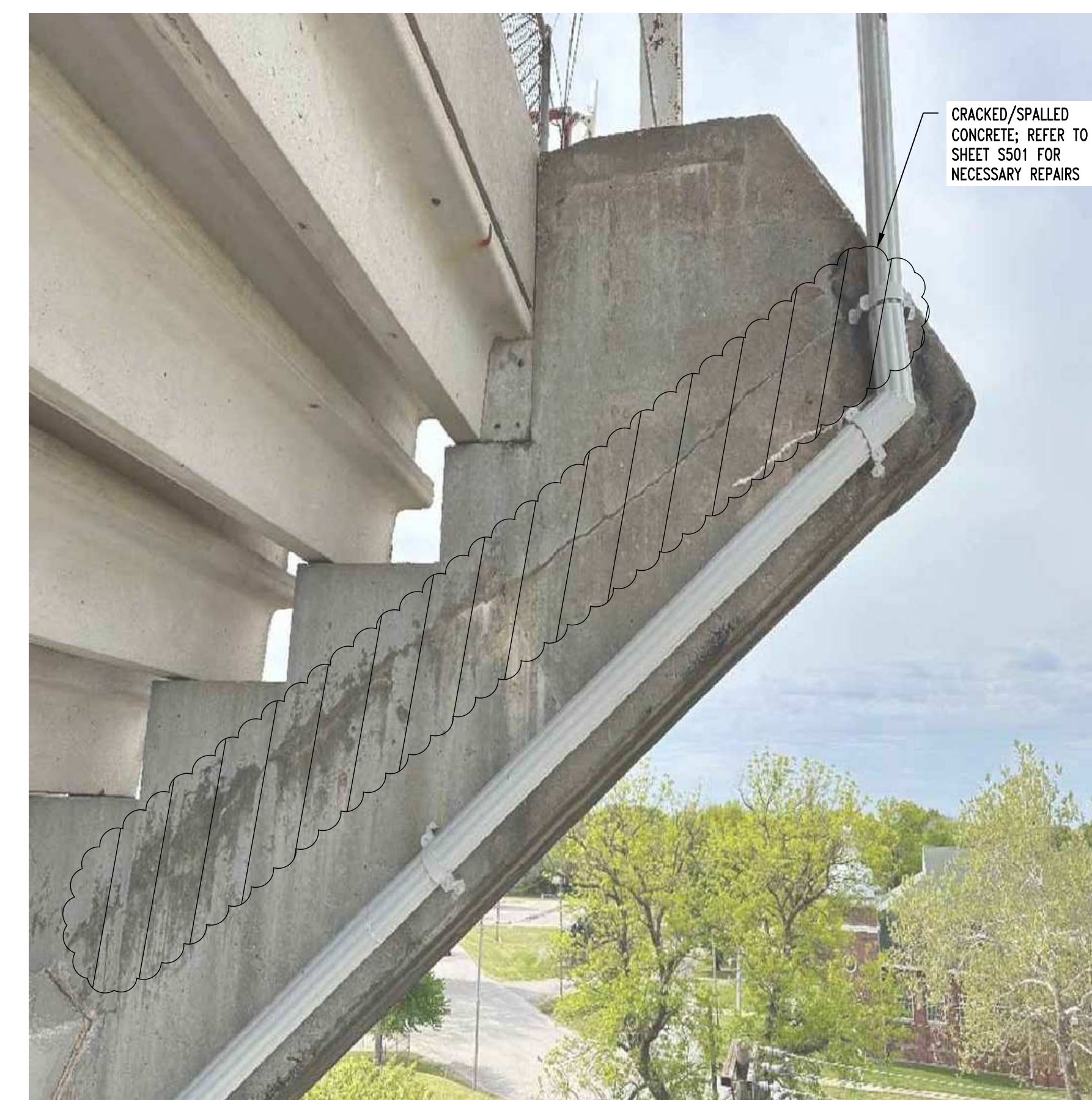
CONCRETE SUPPORT AT GRID LINE 4 (SOUTH FACE)
