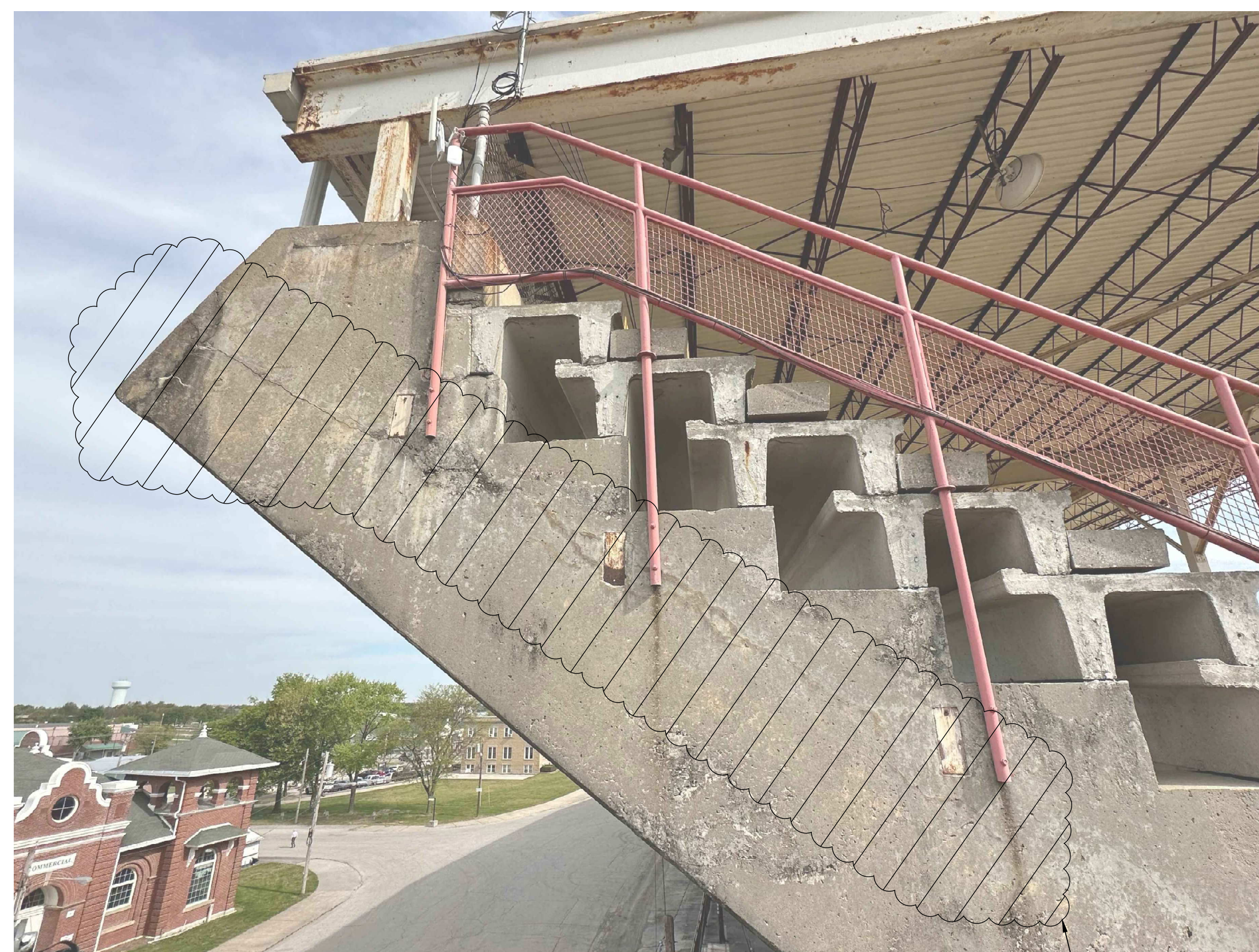
CONCRETE SUPPORT AT GRID LINE 4 (NORTH FACE)
