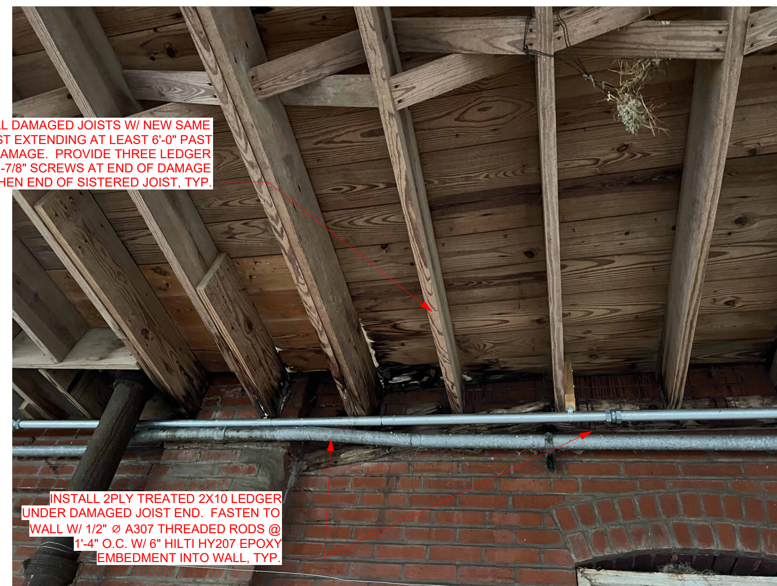
3 STRUCTURAL DETAIL 3 A-508 3/4" = 1'-0"
