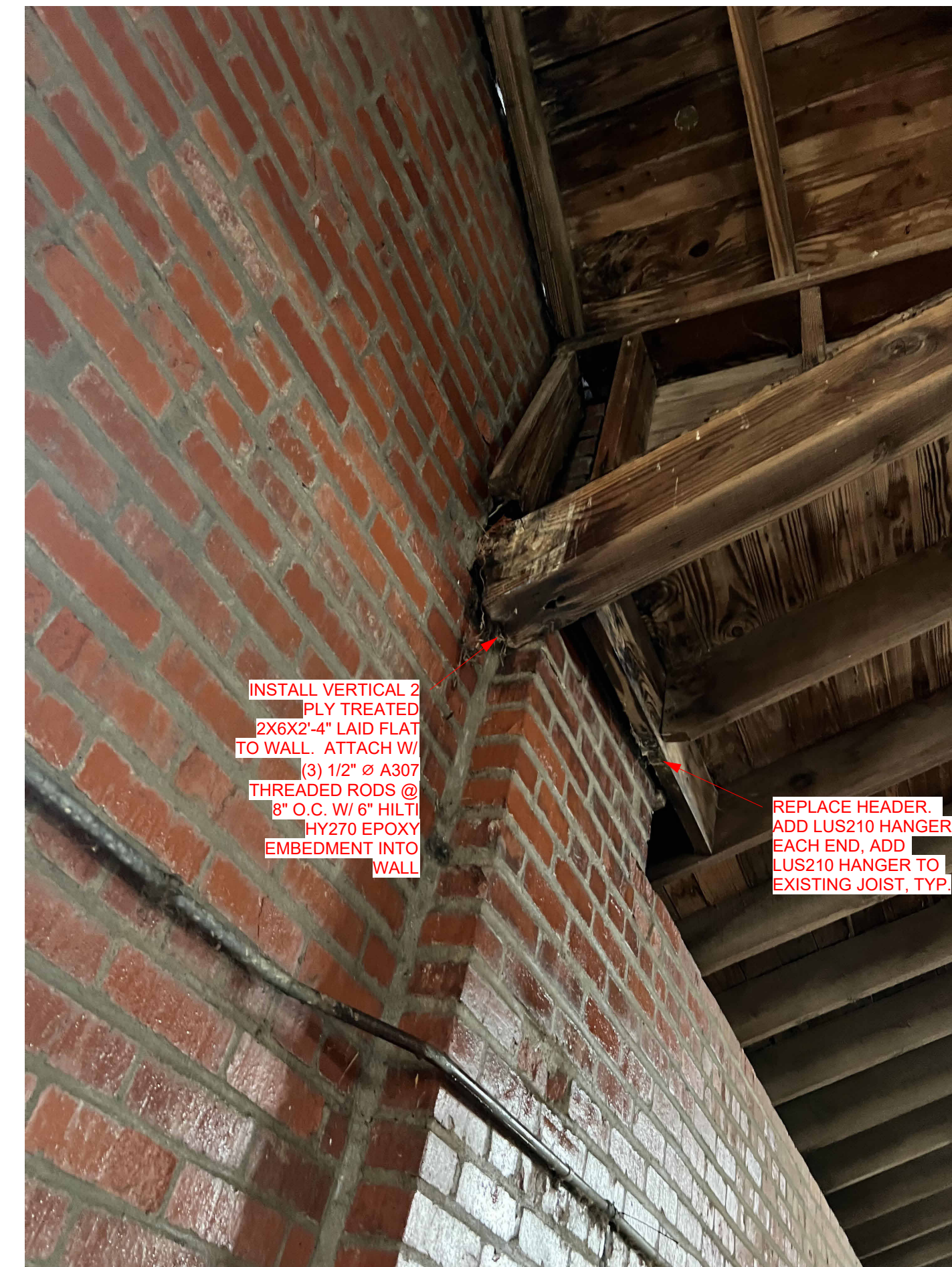
2 STRUCTURAL DETAIL 2 A-508 3/4" = 1'-0"
