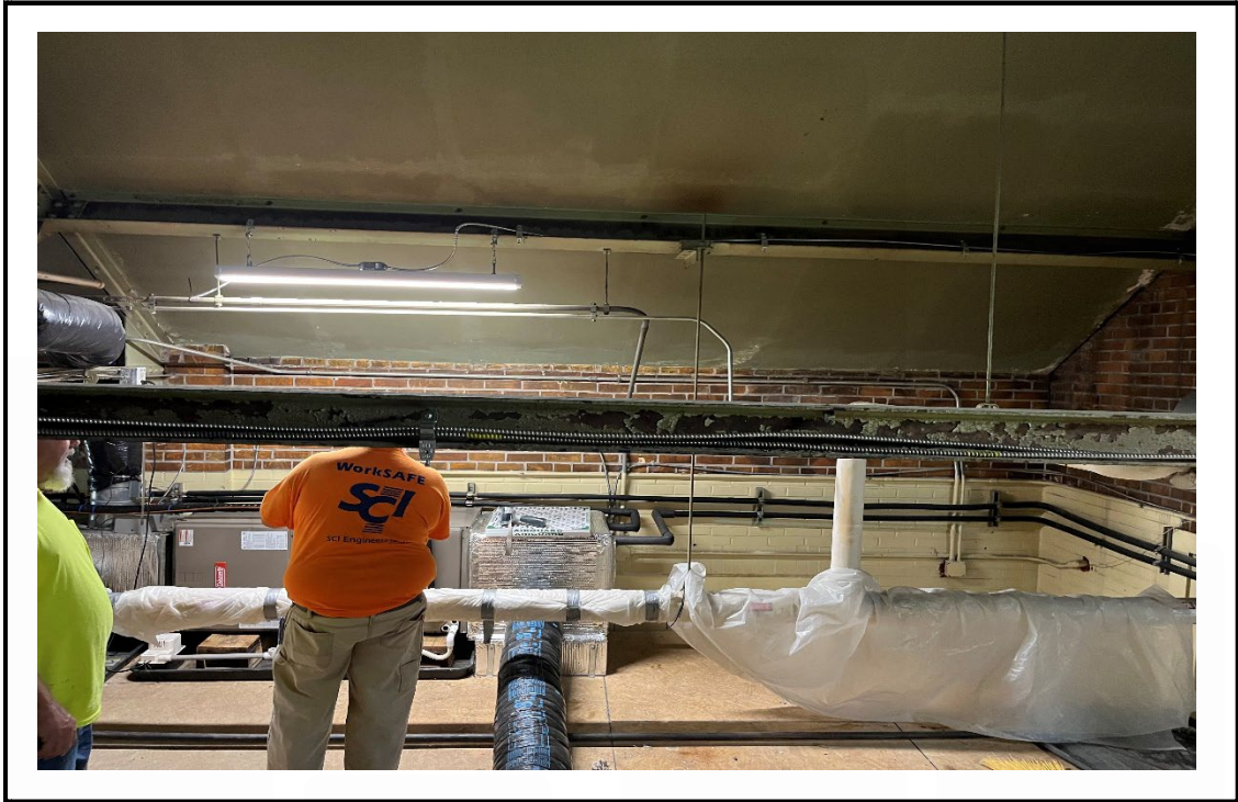
Photo 1. View of the gray metal beam in the Industries Building (Sample 37).
