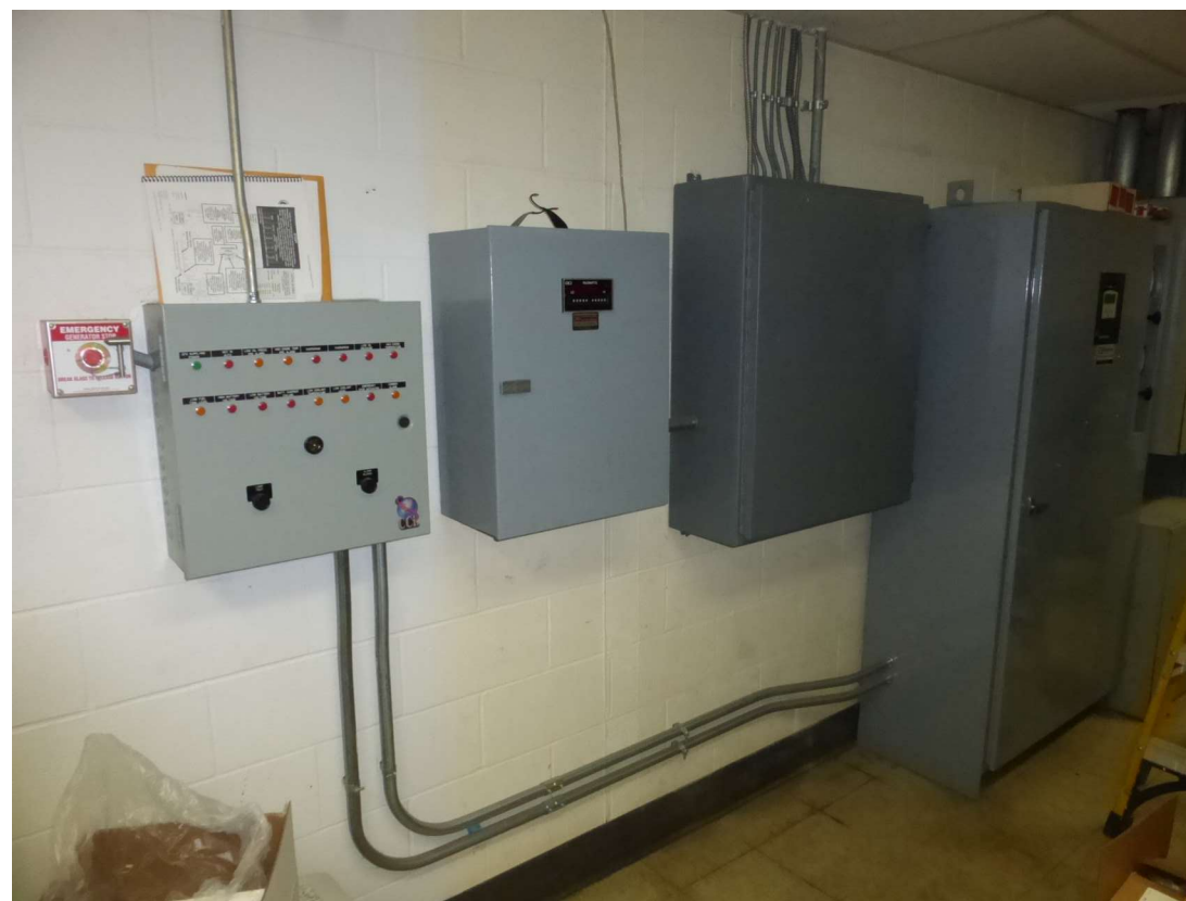
PHOTO 1: ETBR GENERATOR CONTROLS
