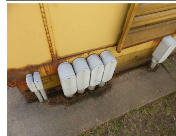
PHOTO 12: ETBR GENERATOR STUB-UPS
