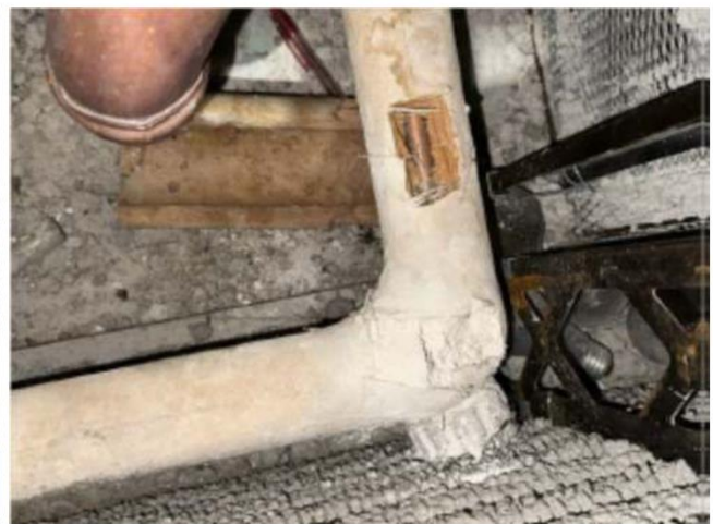
Small Restroom (East) Hard Muddled Fittings 1 & Pipe Insulation 1
