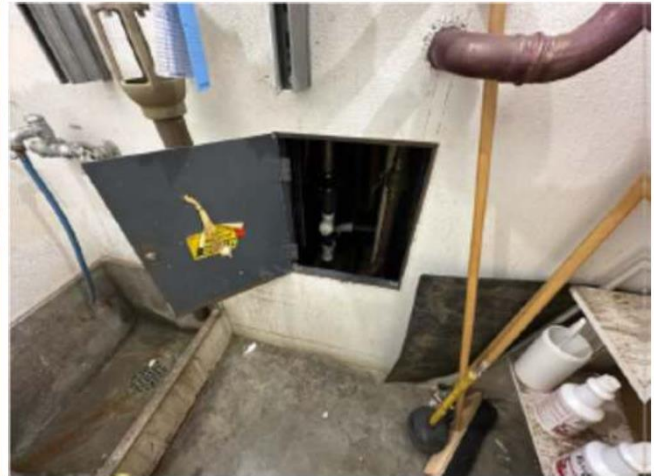
Small Restroom (East) Wall Cavity Access Hatch
