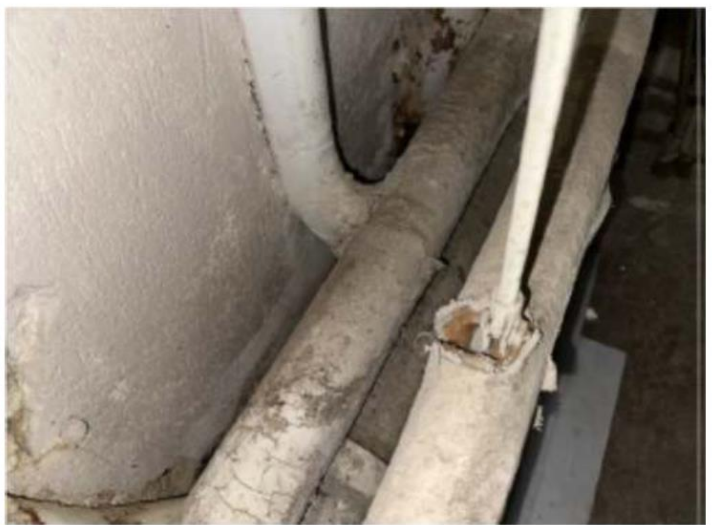
Mechanical Room Hard Muddled Fittings & Pipe Overviews
