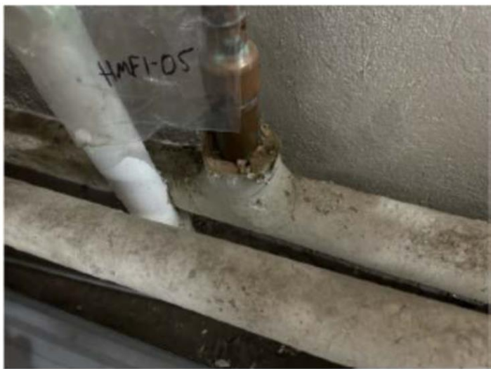
Mechanical Room Hard Muddled Fittings & Pipe Overviews
