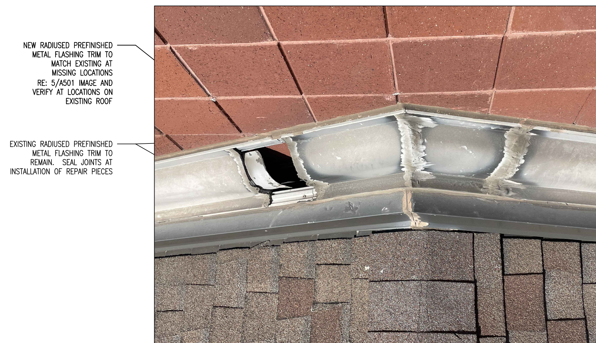
5 EXISTING FLASHING REPAIR IMAGE NTS
