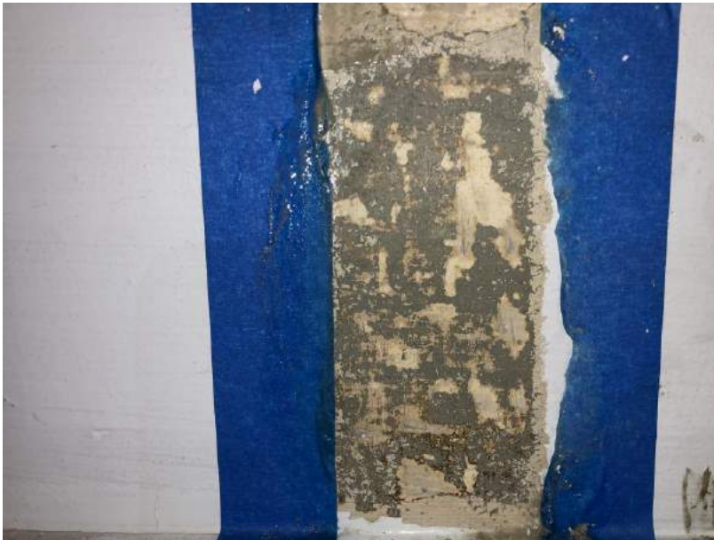
Exposure of the dark green at the cove ceiling.
