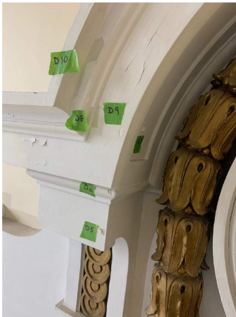
Sample extraction locations (D5-D10) from the entry header.
