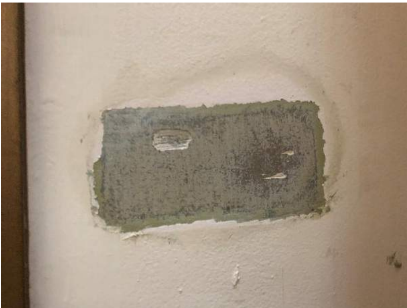
Exposure at the West Wall cove panel.
