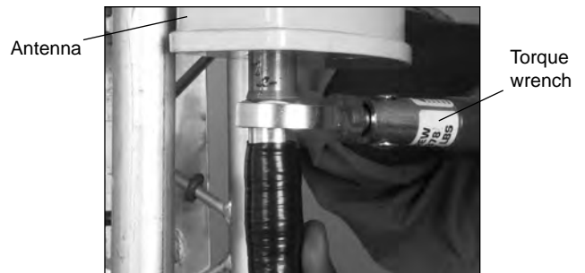
Tighten connection
