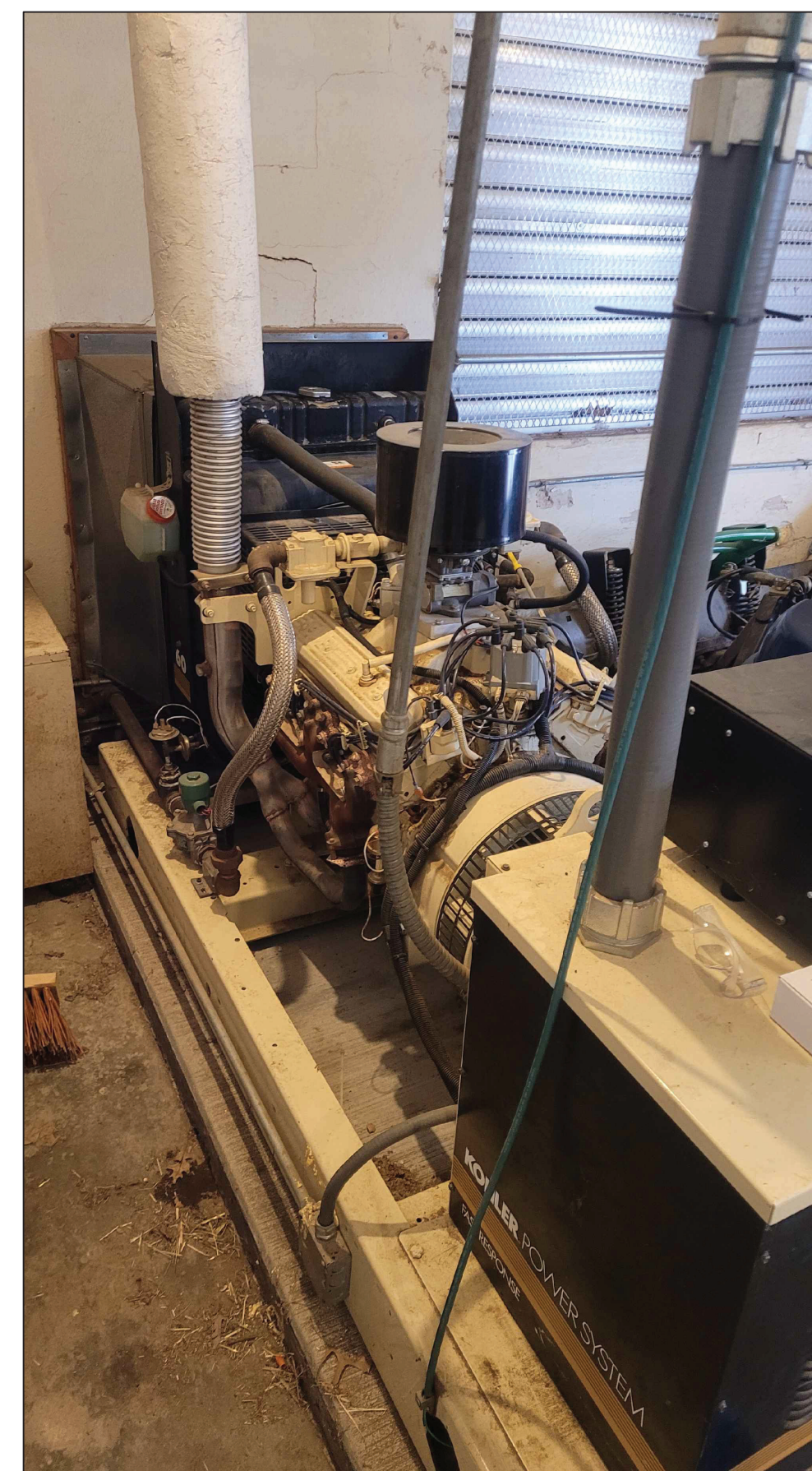
Existing Conduits in Transclosure 5 No Scale E-3
