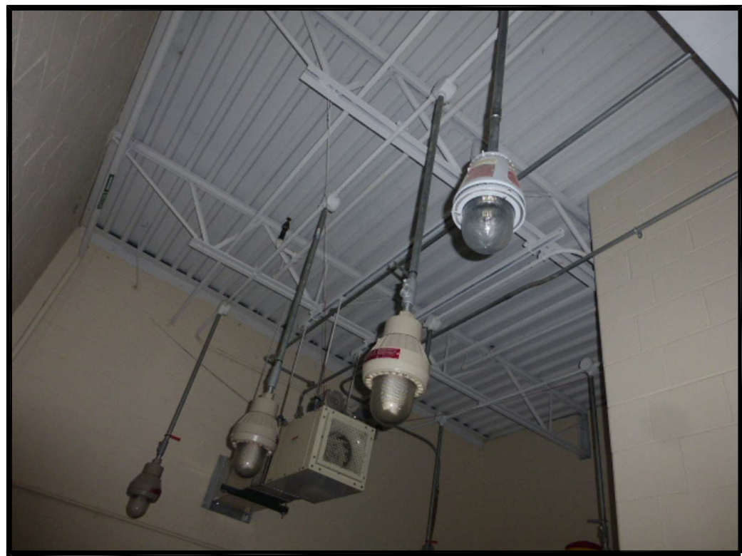
1 TYPICAL EXPLOSION PROOF "N1" AND "R1EM" FIXTURES E101M SCALE: NO SCALE
