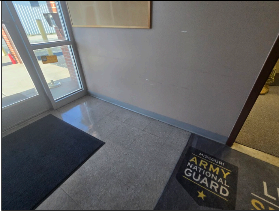
Description: Floor Tile & Mastic
