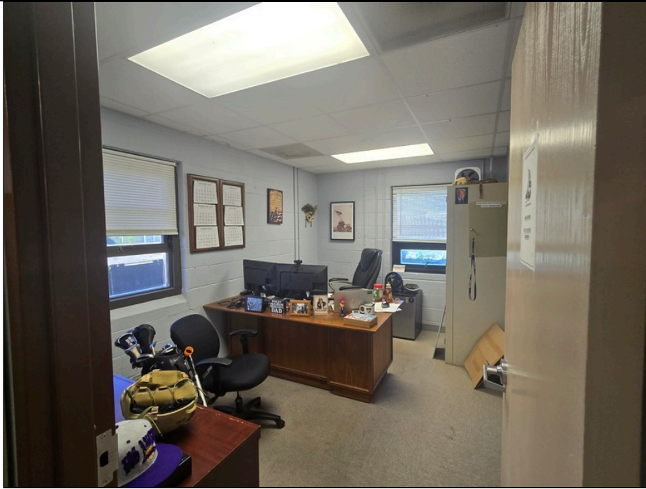
Description: Front offices with mastic under carpet
