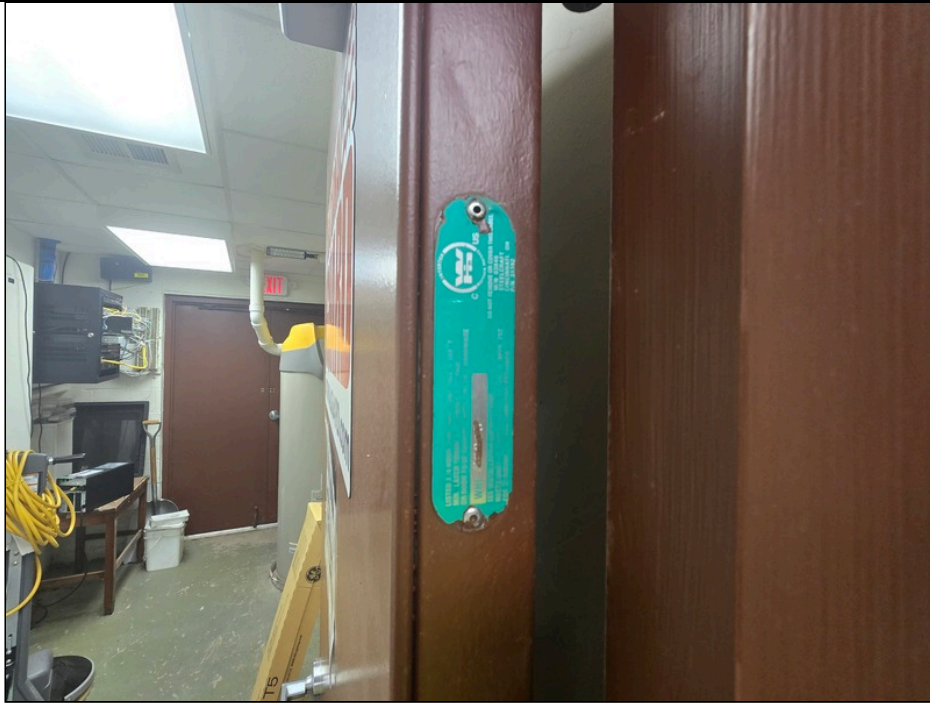
Description: Fire Doors - Assumed
