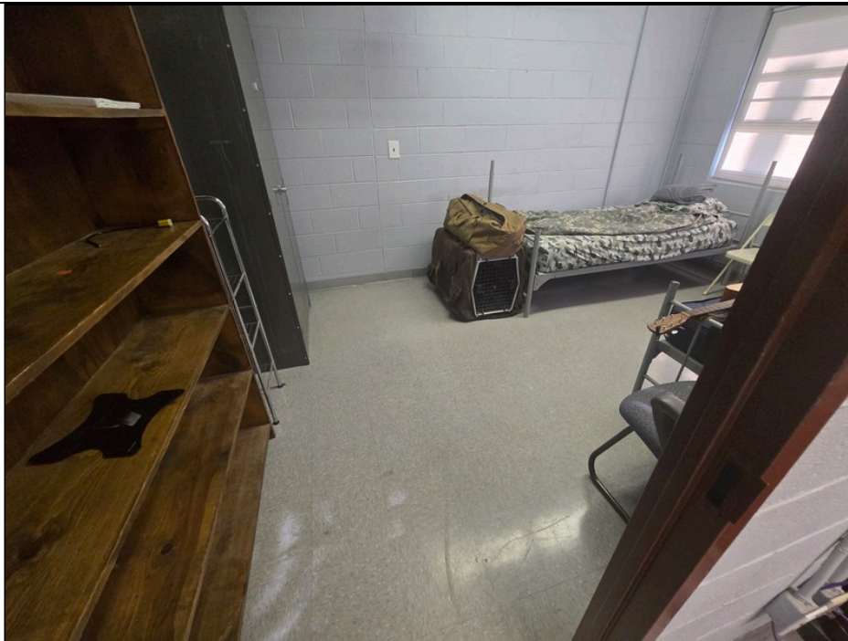
Description: Floor Tile & Mastic
