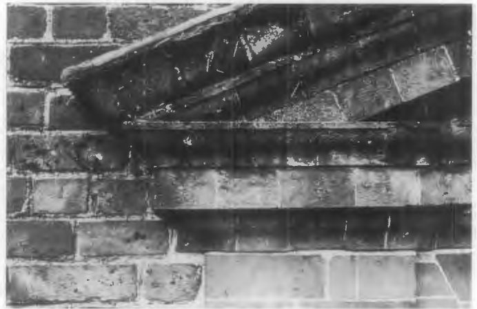
Figure 19. Mortar joints of 18th century brick buildings were often as much as 1/2 inch wide, cut flush and struck with a grapevine joint, but for window and door surrounds where a finer quality rubbed brick was used, mortar joints were very thin. Photo: National Park Service Files.
