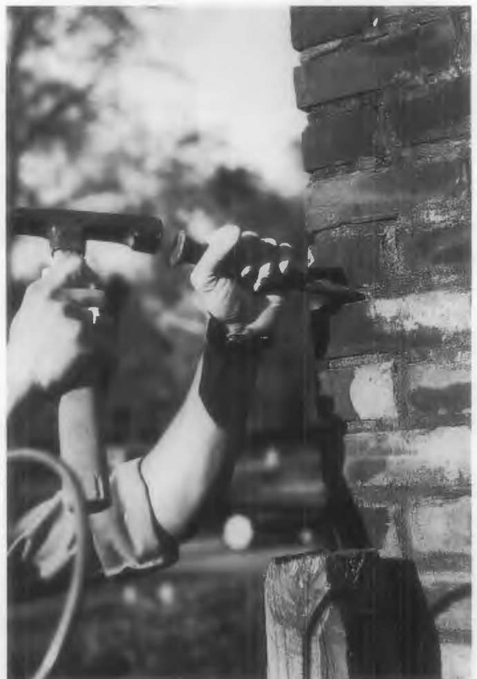
Figure 10. Using a hammer and masonry chisel is the least damaging and, thus, generally the preferred method of removing old mortar in preparation for repointing historic masonry. Photo: John P. Speweik.
