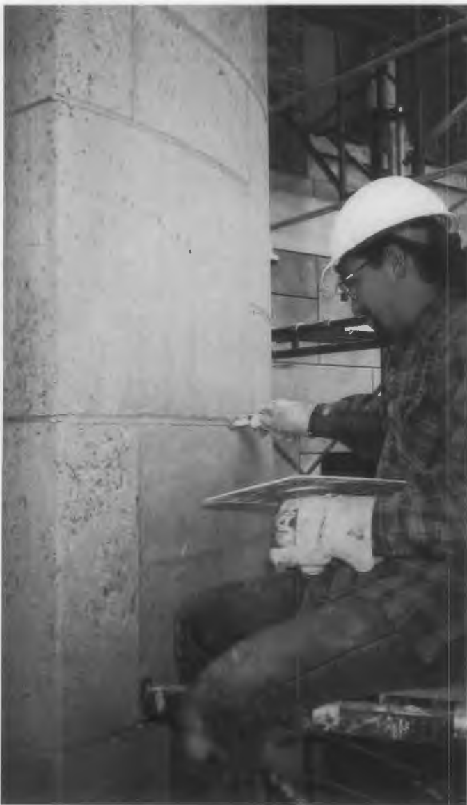
Figure 1. After removing deteriorated mortar, an experienced mason repoints a portion of this early-20th century limestone building. Photo: Robert C. Mack, FAIA.
