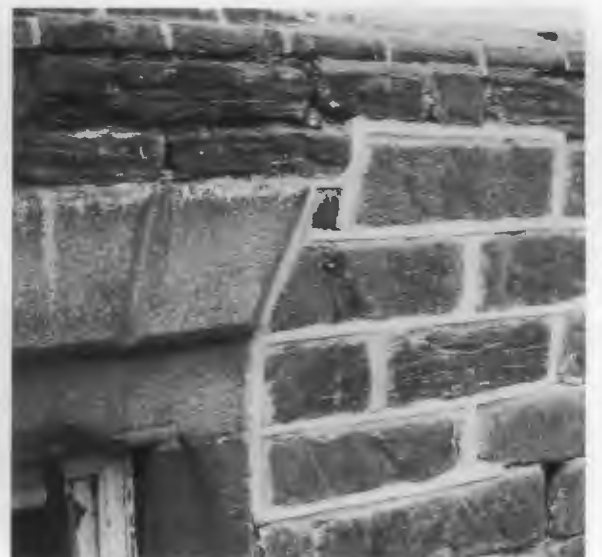
Figure 4. (left) The poor quality of this repointing—it appears to have been “tooled” with the mason’s finger—does not match the delicacy of the original beaded joint on this 19th-century brick wall. (right) It is obvious that the repointing on this “test patch” is not an appropriate replacement mortar joint for this early-19th century stone foundation. Photos: Lee H. Nelson, FAIA.
