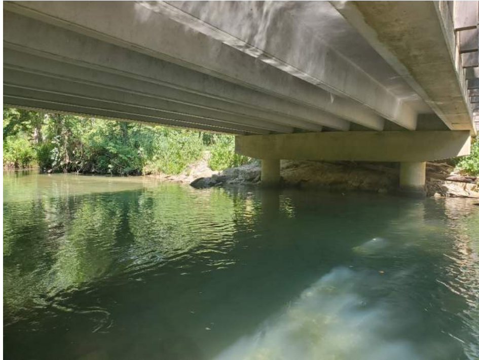
Figure 8: Bridge 3 – Looking east at bottom of bridge
