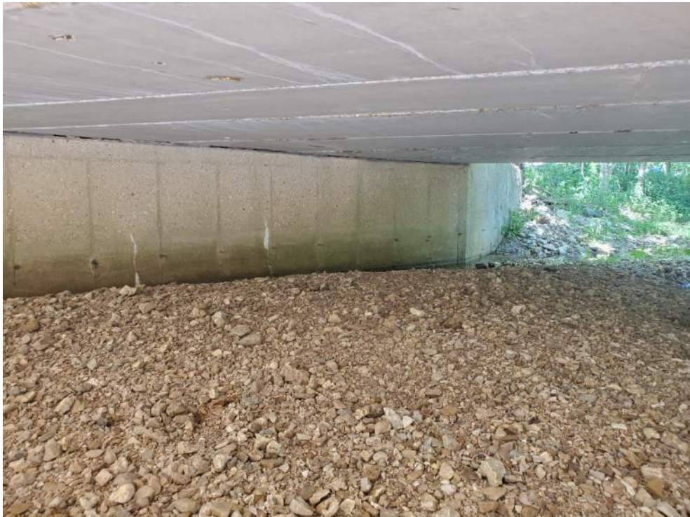
Figure 11: Bridge 4 – Looking east along underside of bridge
