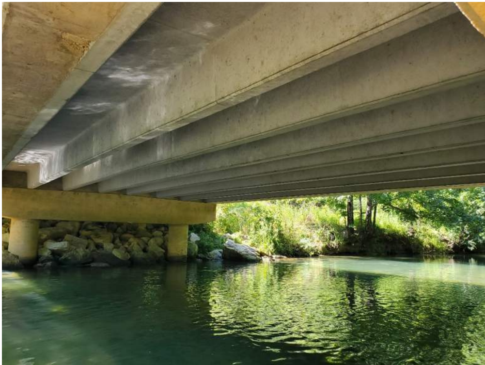
Figure 7: Bridge 3 – Looking west at bottom of bridge
