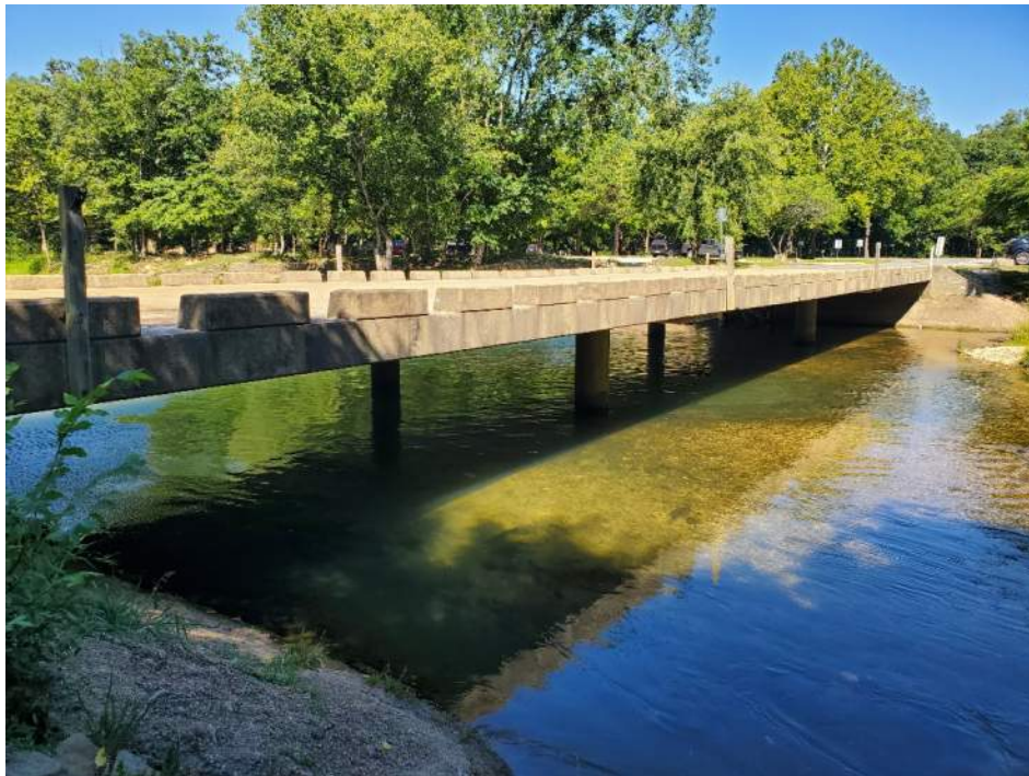
Figure 3: Bridge 1 Elevation View – Looking upstream/NE at fascia
