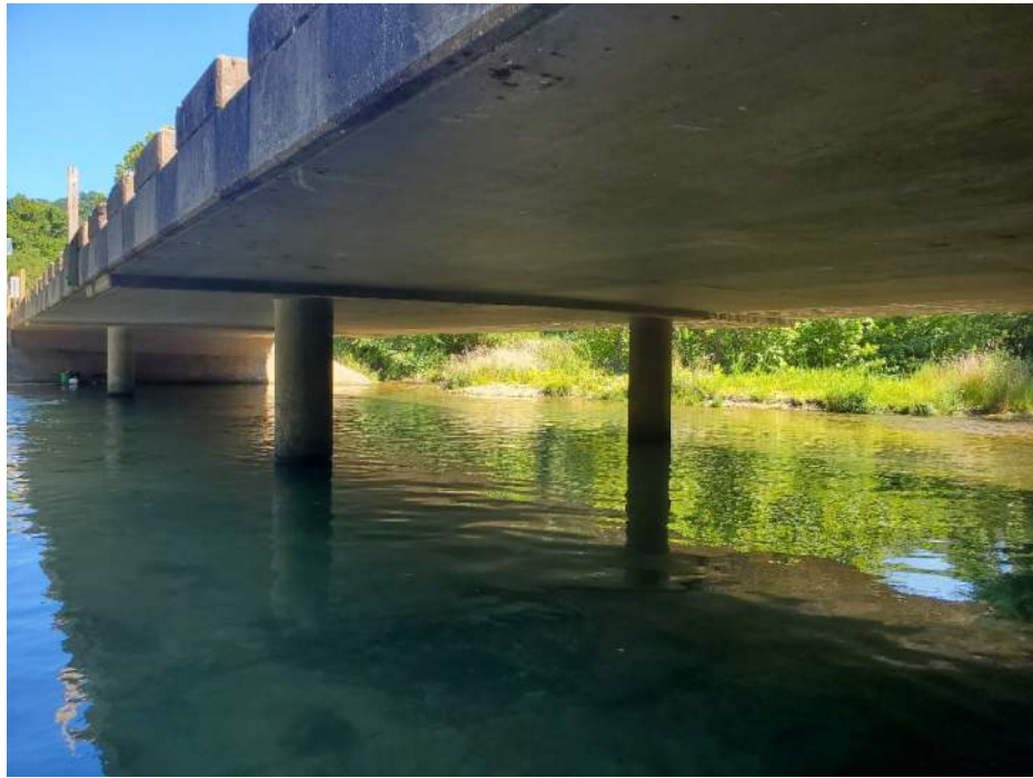
Figure 4: Bridge 1 – Looking downstream/SE at underside of slab
