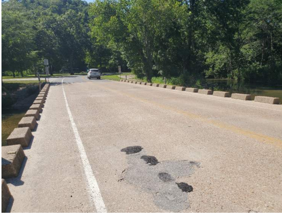
Figure 2: Bridge 1 Deck View – Minor patching visible in deck
