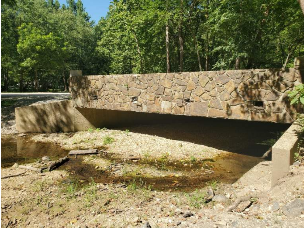
Figure 10: Bridge 4 – Looking east at bridge fascia
