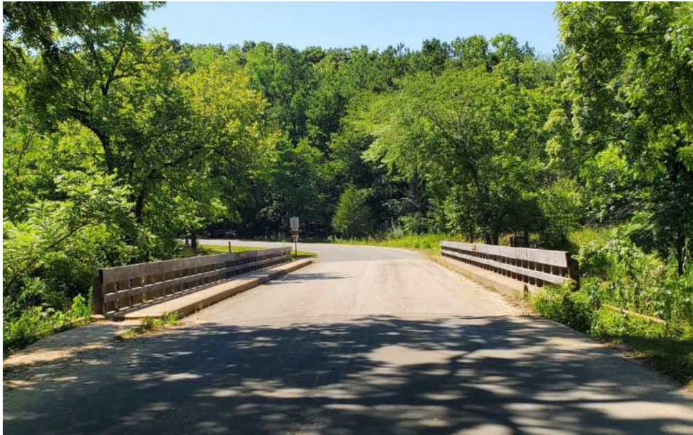
Figure 6: Bridge 3 – Looking west at deck/roadway
